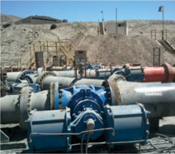
Large diameter DeZURIK PEC Valves in a tailings application
