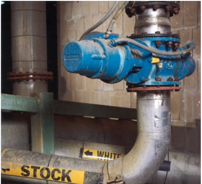
DeZURIK's Precision Electric Basis Weight Control Valve is specifically designed for critical paper stock control, and is used for basis weight and head box level control applications.
