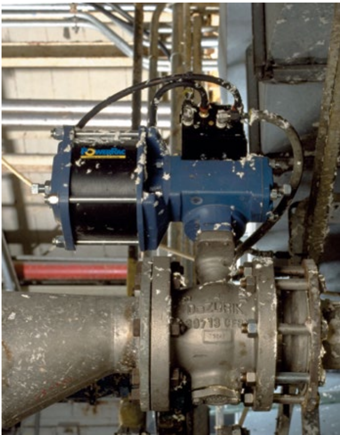
DeZURIK's versatile VPB V-Port Ball Valves are designed for highly accurate control of paper stock, in addition to other clean, dirty or corrosive liquids and gases.
