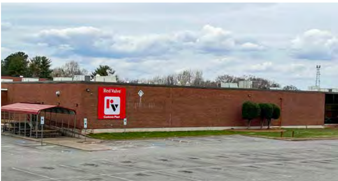
Red Valve Manufacturing Facility, Gastonia, NC USA 155,000 sq. ft.
