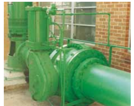
Hydraulic Water Cylinder Actuated List 26
