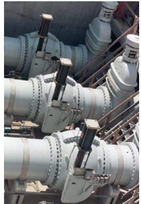
Pump Station Application Air/Oil Tandem Cylinders
