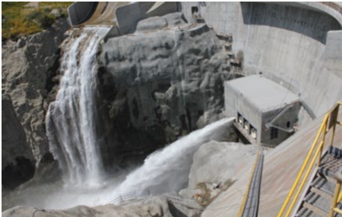
A Hilton 24" Jet Flow Gate (150 psig rating) with motor operator on a dam in Southern California.
