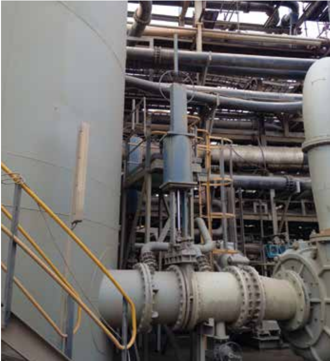
An ASME Pressure Class Severe Service Knife Gate valve in a slurry concentrate pump suction application.
