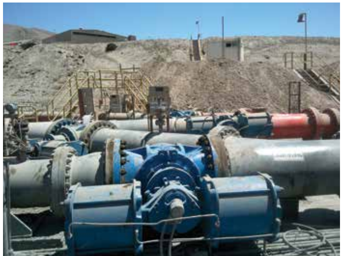
A 24" Rubber Lined Eccentric Plug Valve on a tailings application.
