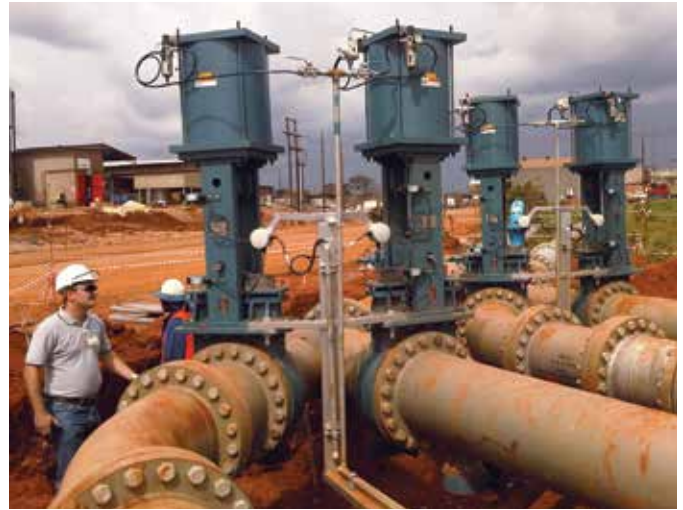
Four ASME Class Severe Service Knife Gate Valves in slurry service at a copper mine.
