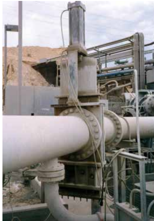
A 30" Bonnetless Thru-Port Gate Valve in Carbon Steel construction with Tungsten-Carbide Hard Faced Gate and hydraulic cylinder in abrasive slurry service.
