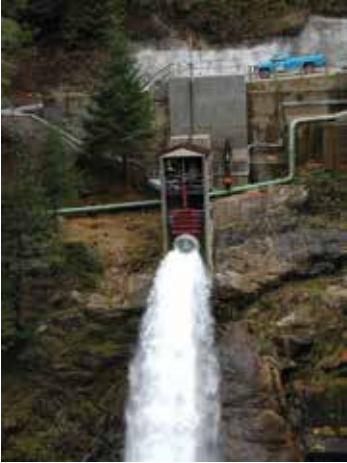
A 48"/60" Hilton Throttling Knife Gate Valve (50 psi rating) with electric motor operator is installed on a flow modification project.
