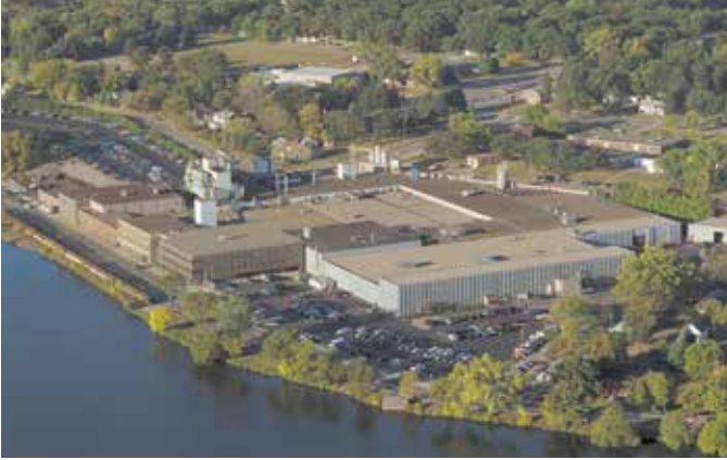
DeZURIK Corporate Headquarters and Manufacturing facility, Sartell, MN USA. Established in 1928, 420,000 sq. ft.
