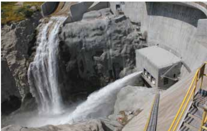
A 24" Jet Flow Gate (150 psi rating) with motor operator on a dam in Southern California.
