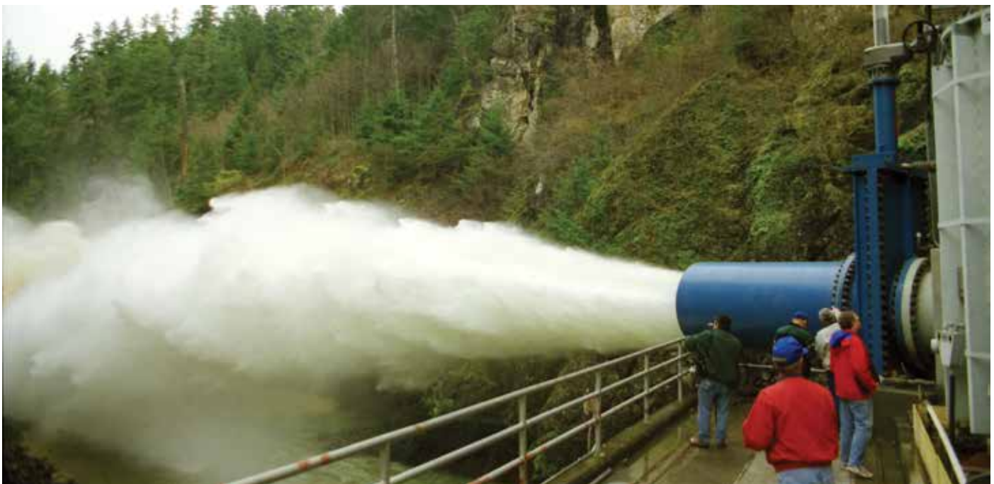
This 42" Hilton Jet Flow Gate Valve is installed at LaGrande Dam near Tacoma, Washington.
