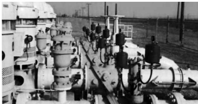
Top mounted valves are excellent for vertical turbine pumps without a Variable Frequency Drive.
