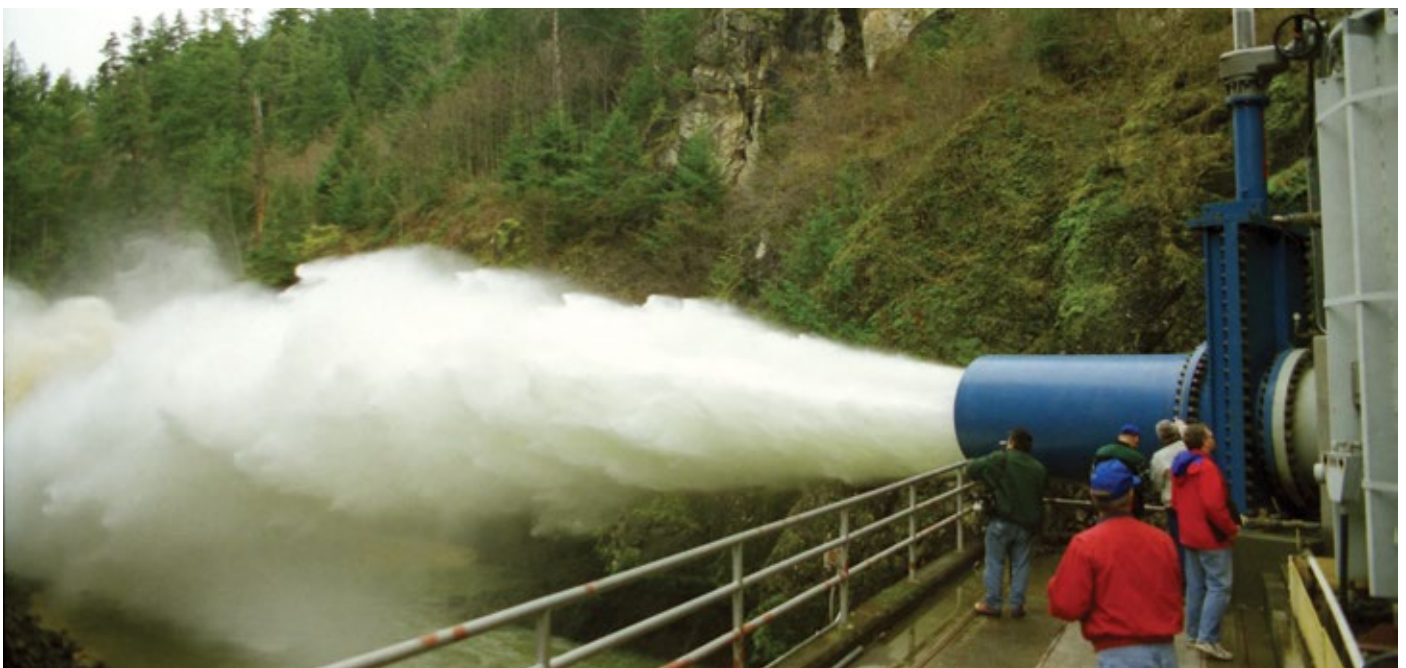
This 42" Hilton Jet Flow Gate is installed at LaGrande Dam near Tacoma, Washington.
