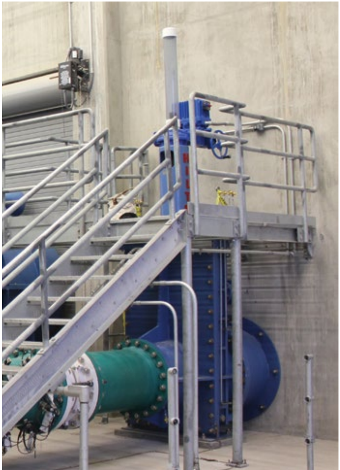
A Hilton 24" Jet Flow Gate (150 psig rating) with motor operator on a dam in Southern California.
