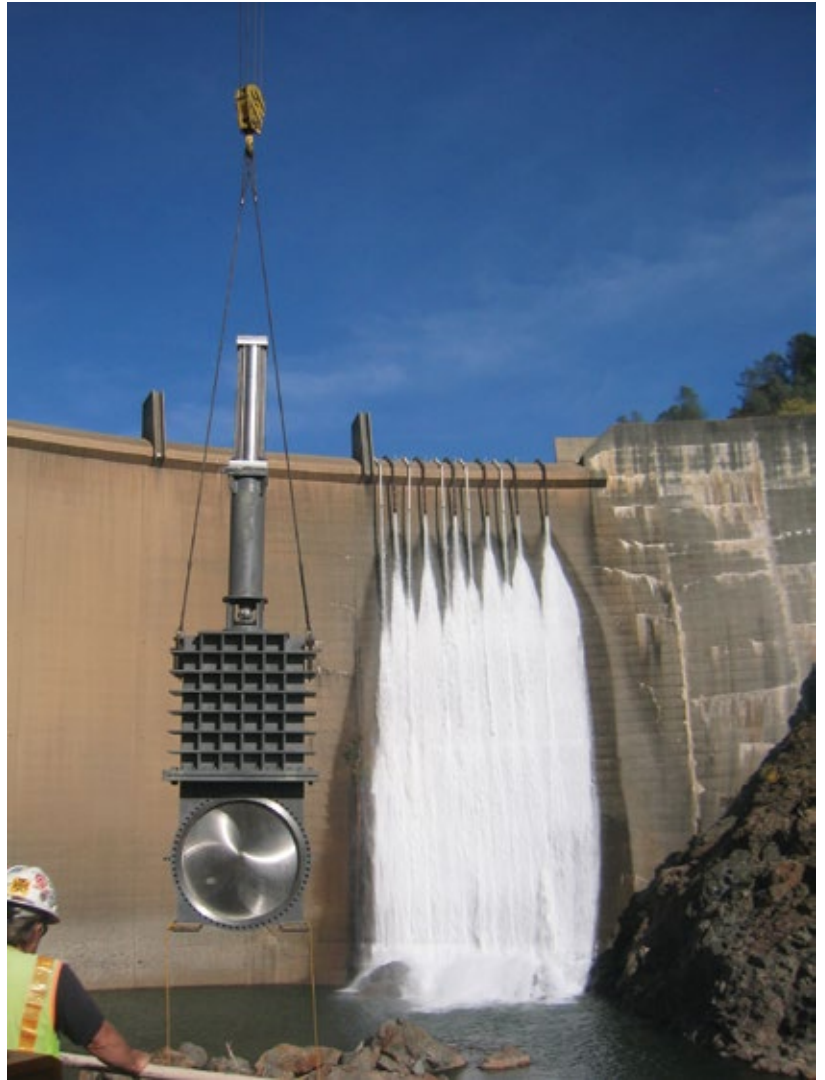
A 72" Hilton Bonneted Knife Gate Valve (130 psi rating) with hydraulic cylinder actuator is used for a guard valve for a Fixed Cone Valve at a dam in northern California.
