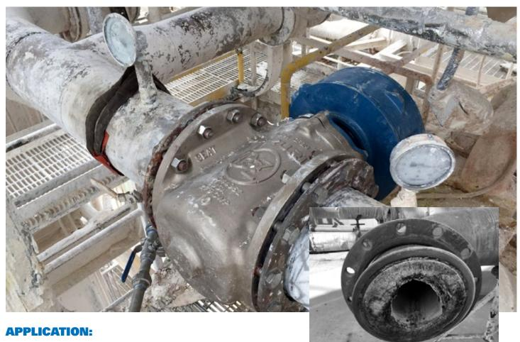
A pulp and paper mill was experiencing routine operational challenges when isolating a green liquor process due to a failing tapered plug valve. The 12" tapered plug valve was used to stop the flow of green liquor so that scheduled maintenance could be performed on the process slaker. Operators often used a 12' long bar inserted in the actuation mechanism to break the valve from the open position and close it.
