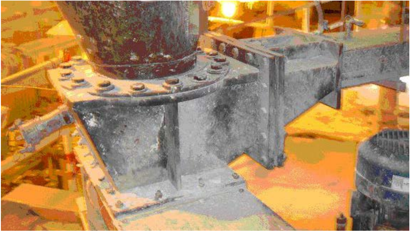
The Hilton Material Handling Knife Gate Valve, with a fabricated displacement pocket and bonnet, is designed to operate against a standing column of dry, packed material.
