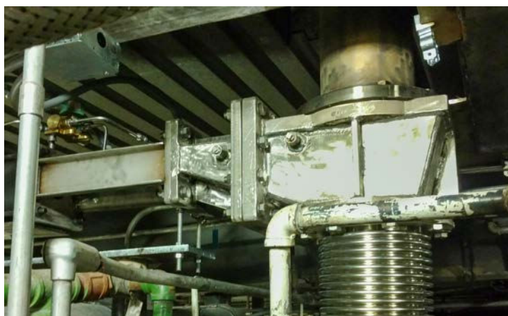
Hilton Material Handling Knife Gate Valve with Bonnet installed in a power plant on a hot bottom ash application.
