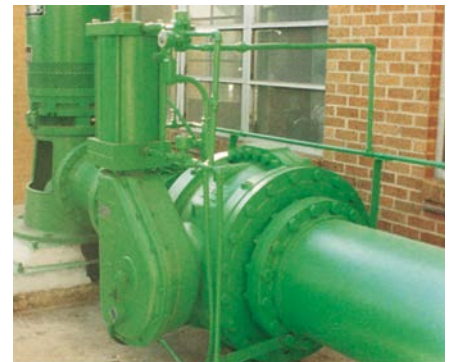
Hydraulic Water Cylinder Actuated Metal Seated Ball Valve
