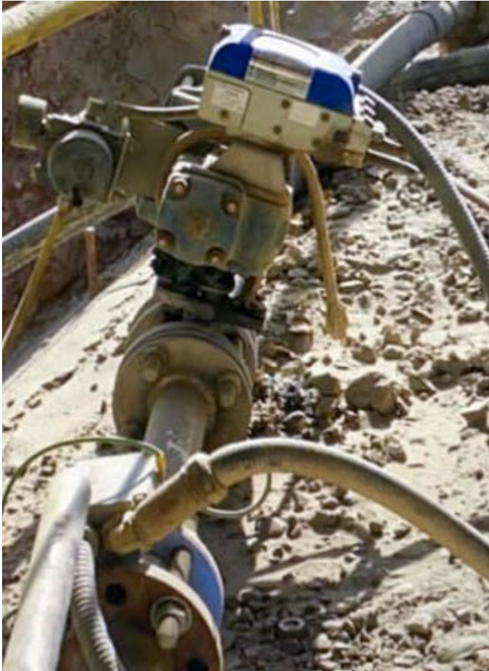
Field installation of 2" RCV for raffinate control
