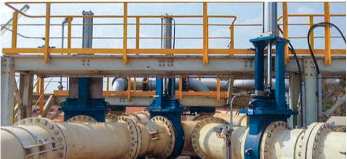
DeZURIK KSV Severe Service Knife Gate Valves installed in a tailings slurry pump isolation application. The KSV valves lasted 14 times longer than the push through style valves in this challenging service.
