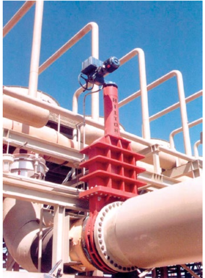
This Hilton 42" Bonneted Knife Gate Valve is installed at a Geothermal plant in the Western United States.
