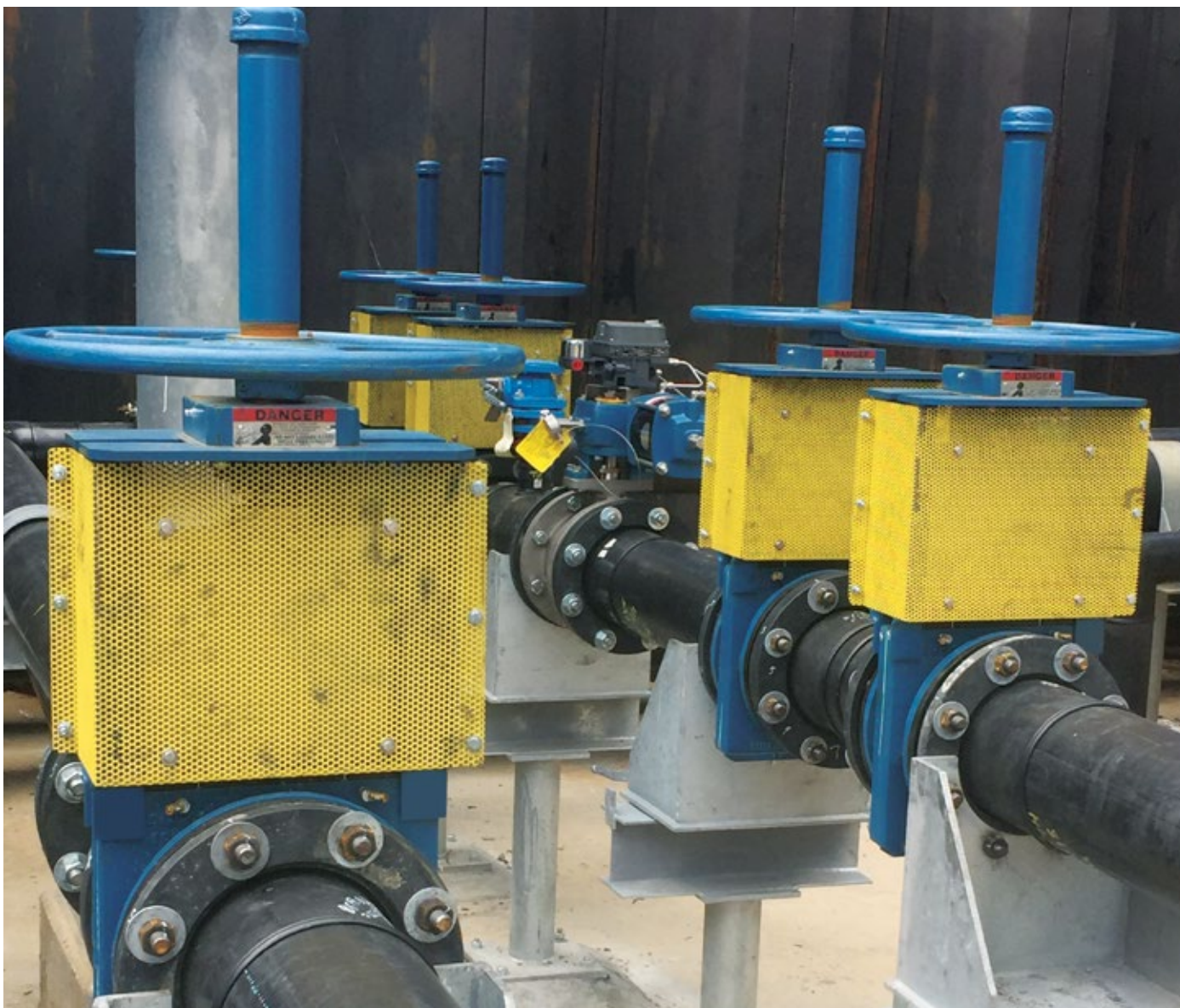
DeZURIK KSL Slurry Knife Gate Valves equipped with optional gate guards on a FGD return water system.
