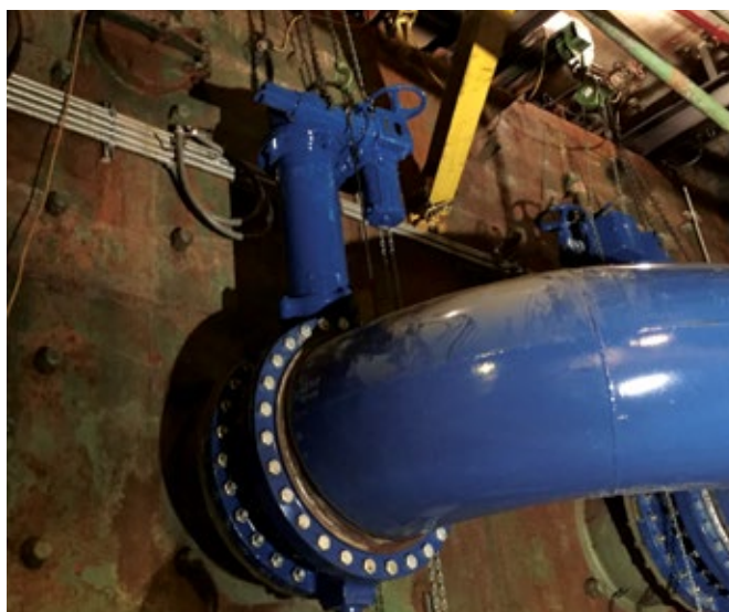
DeZURIK AWWA Butterfly Valves with neck extensions and electric motor actuators isolate water to the condenser.
