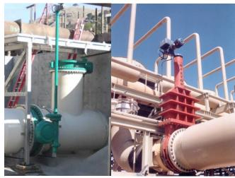
**H-200B Hilton Bonneted Knife Gate Valves** are engineered and fabricated to meet the most challenging corrosive conditions. Fully welded body liner options utilizing multiple alloys including Monel, Hastelloy and various grades of stainless steel. Size ranges to 144".
