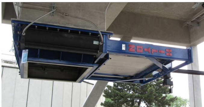
Material handling knife gate valve on the bottom of a hopper.
