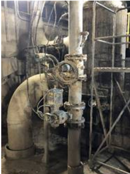
6" DeZURIK V-Port Ball Valve (VPB) with Recycle Reject Trim Package, PowerRac actuator and PMV positioner controls the flow of rejects from the pressure screen to the pulper.
