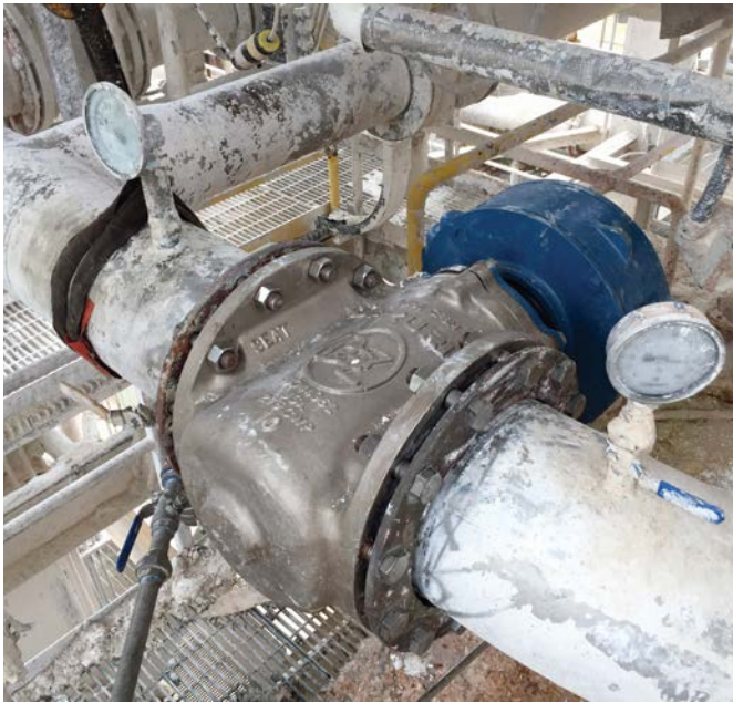
DeZURIK PEC Eccentric Plug Valve in a pulp mill on a green liquor isolation application.
