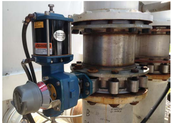
DeZURIK High Performance Butterfly Valves are ideally suited for a wide variety of services including water, steam, liquor and other corrosive liquids and gases.
