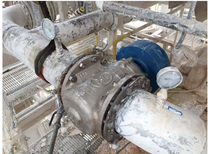
DeZURIK PEC Eccentric Plug Valve in a pulp mill on a green liquor isolation application.
