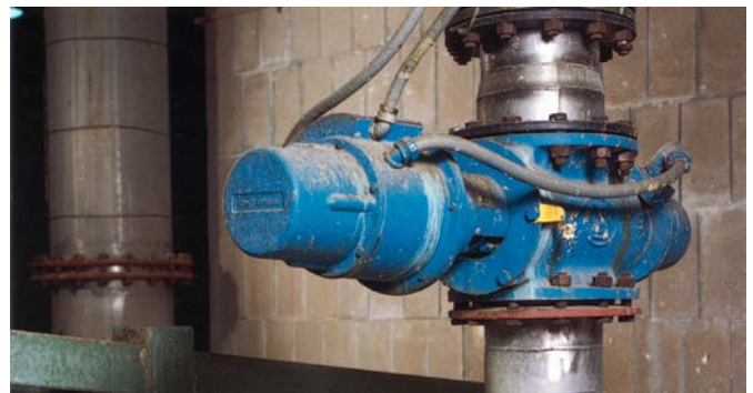
DeZURIK's Precision Electric Basis Weight Control Valve is specifically designed for critical paper stock control and is used for basis weight and head box level control applications.
