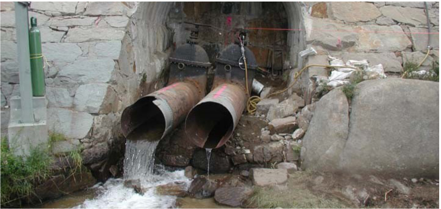
The conventional wedge gate valve was a common outlet valve in the early days of hydro.
