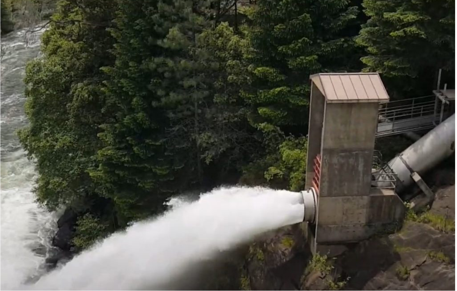
The throttling knife gate valve is an economical outlet valve for low head dams. This 48-in throttling knife gate valve at Tiger Creek Afterbay Dam in northern California satisfies instream flow requirements.
