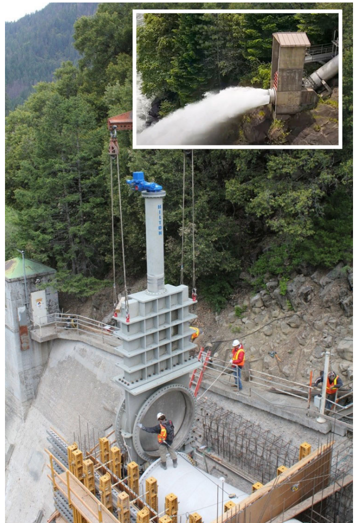
The throttling knife gate valve is an economical outlet valve for many hydro applications.
