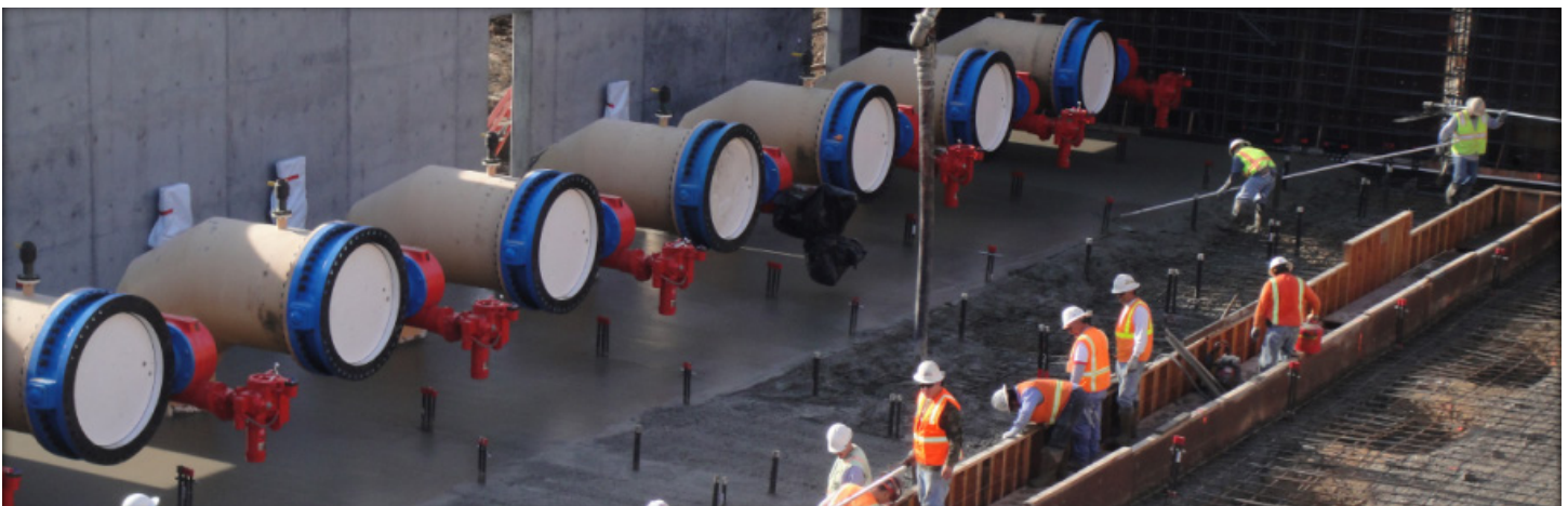
48" AWWA butterfly valves equipped with electric actuators are installed at a water treatment disinfection facility for precise flow control.
